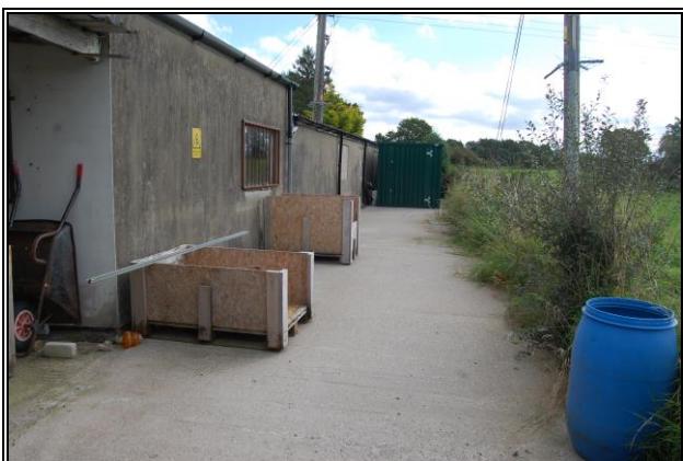
Rear External Storage Area East
